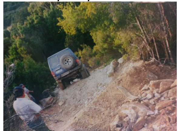
Building a new track, Mt Reid
